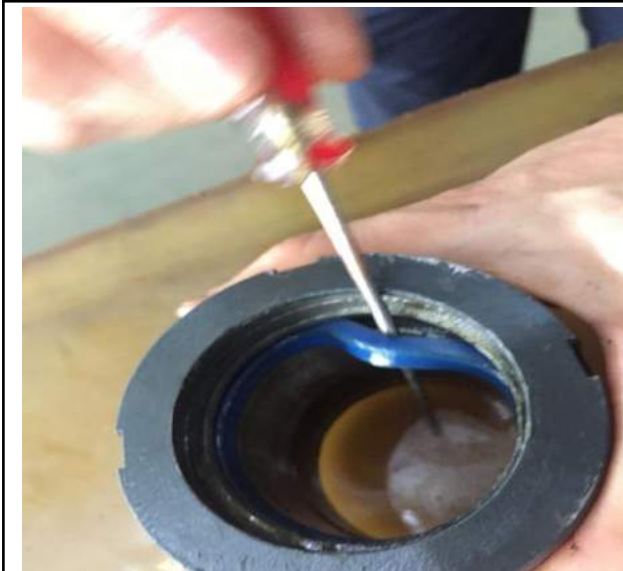
2. Remove dustproof seal and shield ring and Y-type seal
