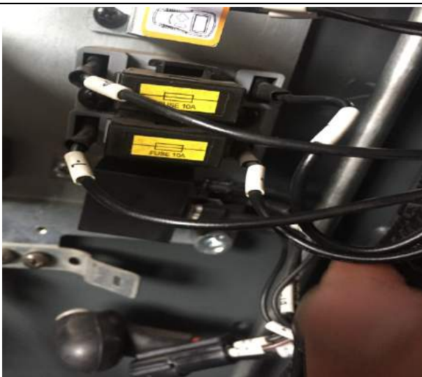
4. Unplug the plug and write down the line number. The position of the line number is shown in the table on
