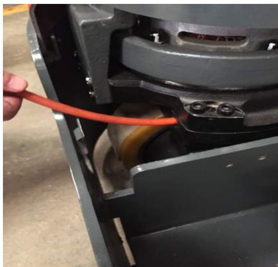
6. Lubricating oil through tubing. The lubricant used is 85W/90 GL-5 heavy duty vehicle gear oil.
